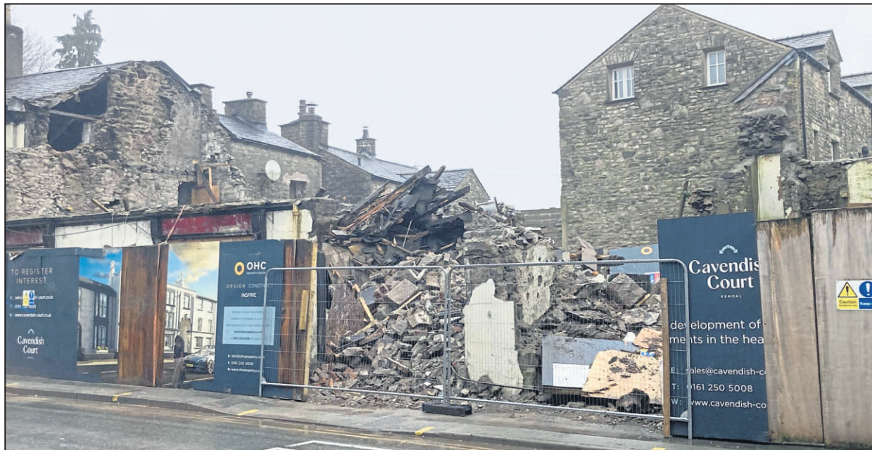
The demolished site on Stricklandgate
