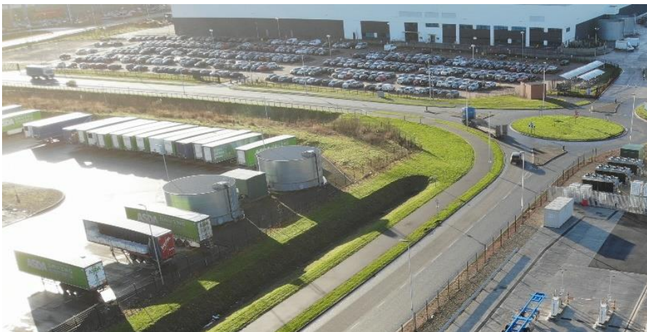
Warrington – the largest bio-CNG refuelling station in Europe
