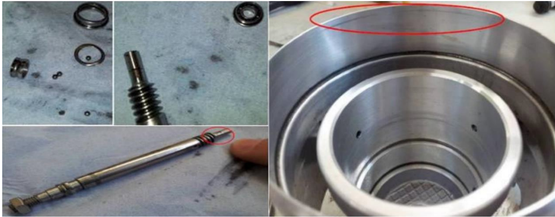
Figure 9: Pictures of the components (ball bearings, turbine shaft and internal wall) that failed at Silk Willoughby
