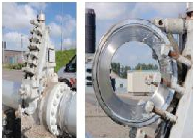
Figure 2: Orifice plate carrier and orifice plate
