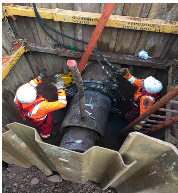
Figures 5 & 6: Pipe/sleeve interaction, and the initial sleeve shortening operation
